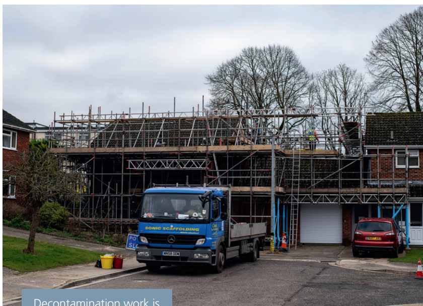
Decontamination work is still being undertaken on the Skripals' residence in 2019
